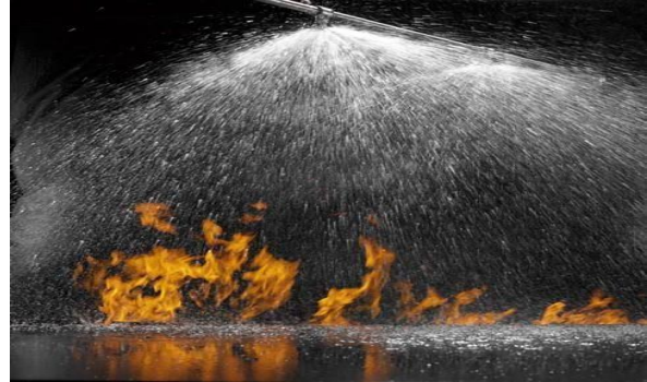
Fig 2: Automatic fire extinguishing sprinkler.
